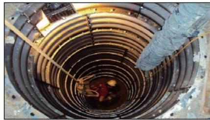
(a) 鋼襯板保護人工挖掘
