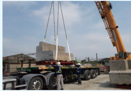
(6)外牆及軌道平臺提取移置
