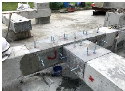
(c) 梁柱接頭補強[51]
